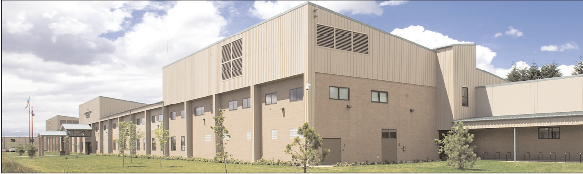
Courtesy of BBL Architects The building constructed during the second phase of the Lane County Armed Forces Reserve Center project in Springfield qualified for Leadership in Energy and Environmental Design gold certification.
